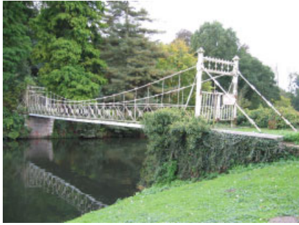
Fig. 5. Current state of the suspension bridge (2003)
