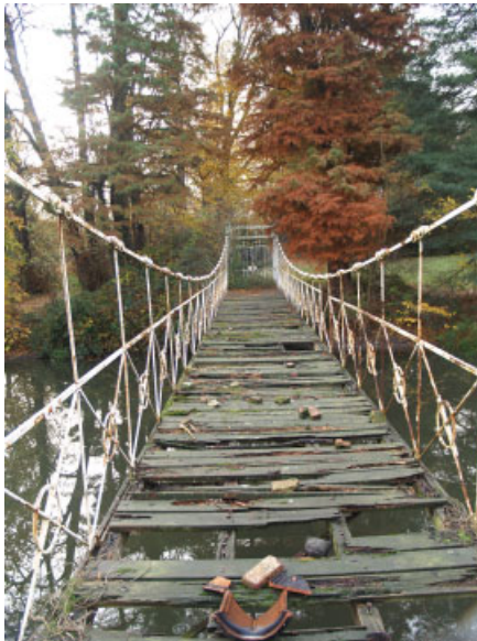
Fig. 6. View of the suspension bridge deck (2006)
