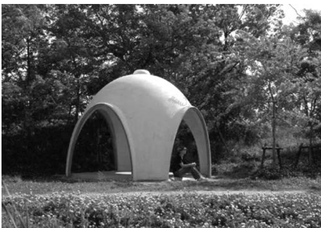
Figure 11. Sakan Shell Structure project, architect Kazuya Morita
