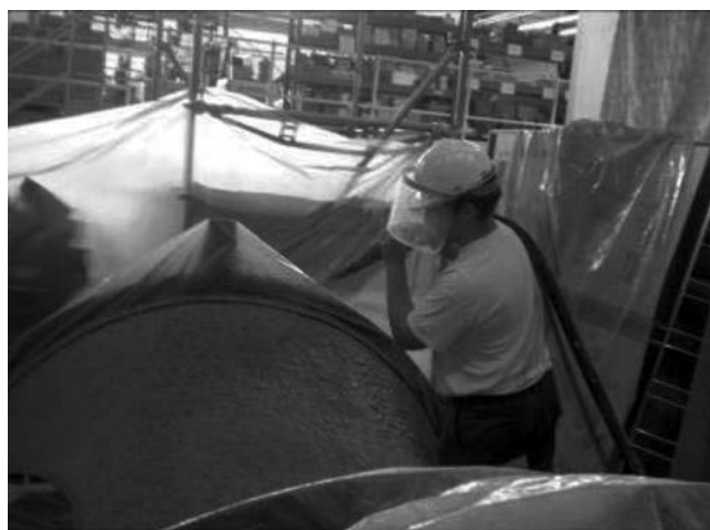
Figure 22. Concreting of the shell on fabric formwork with shotcrete
