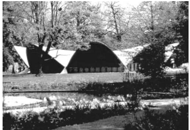
Figure 12. GRC shell by Schlaich, for Federal Garden Exhibition in Stuttgart (Holgate 1997)
