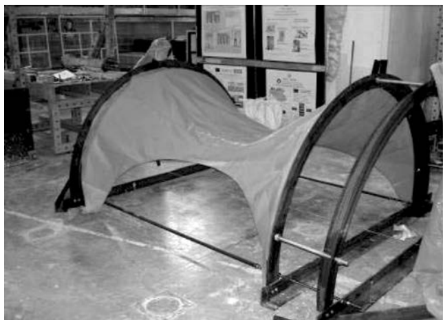
Figure 19. Formwork setup before casting
