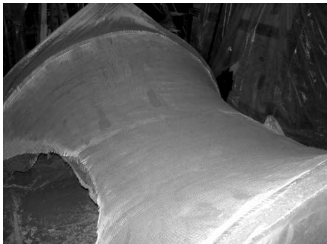
Figure 21. Applying the textile reinforcement
