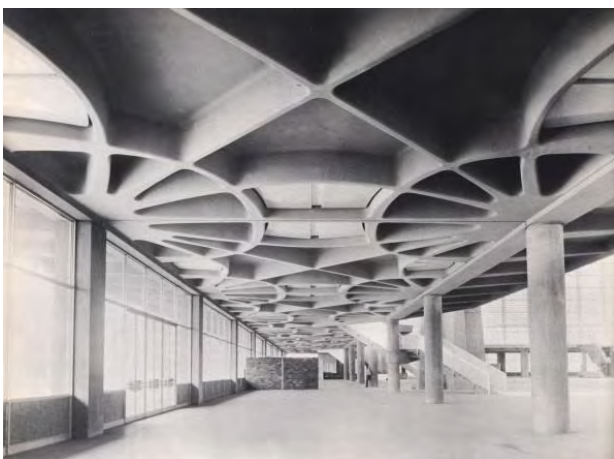
Fig. 7. Palace of Labor Floor System [13]
