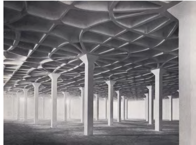
Fig. 4. Gatti Wool Factory Floor System [13]
