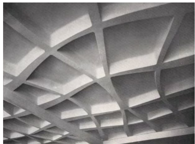
Fig. 9. Large Sports Palace Floor System [25]
