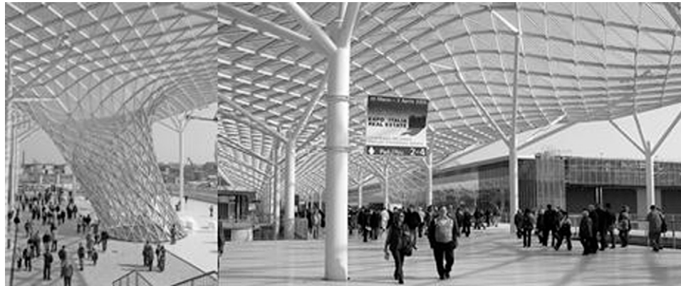
Fig. 2. Nuovo Polo Fiera Milano (Italy, built in 2004; architect Massimiliano Fuksas, structural engineers Schlaich Bergermann and Partner and Mero TSK Group) illustrates how a sculptural shell is discretized in four-sided and triangulated (at the supports) meshes
